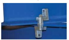
STEP 4 - Ensure the locknut is tightened to the top of GirderFix clamp using the method finger tight plus 1/4 turn.
